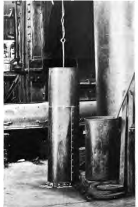
Fig. 2. Counterweight protected by Steel Tube.*
